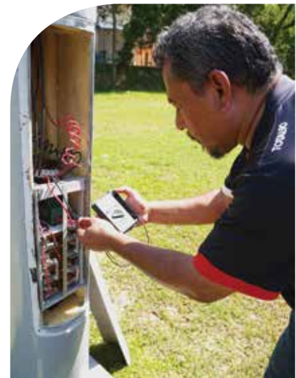
SIRIM Lithium-Ion Battery for the APAIS system
