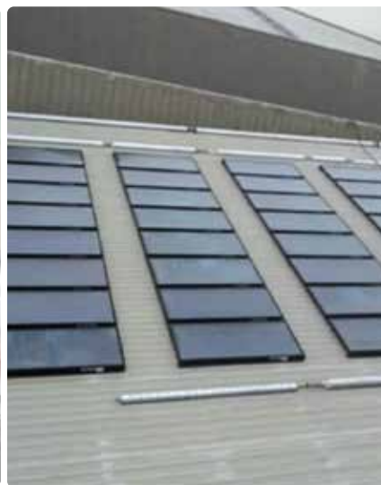
40 PLATE COLLECTORS INSTALLED ON ROOF TOP
