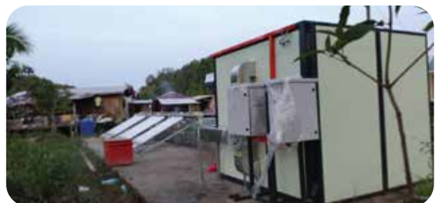
Solar Drying System of tapioca chips
