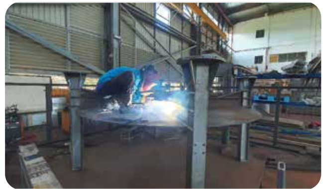
Welding Work of an Ongoing Project
