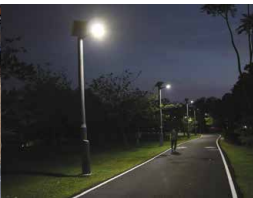
▲ Solar Street Lighting
